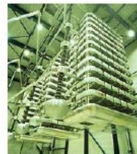
Fig. 3: 150mm PCT rated at 8.5kV/4000A for UHVDC.
